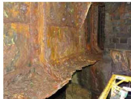
■ The railway bridge at St Margaret's Street/Trowbridge Road is in very poor condition and cannot be economically repaired
