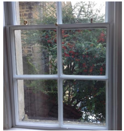
Secondary glazed front window.
