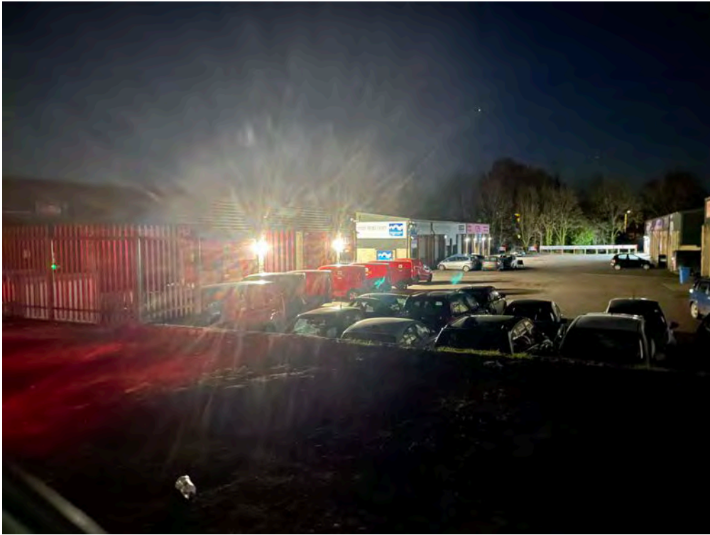
Plate 13. Business / Security Lighting at Treenwood Industrial Estate
