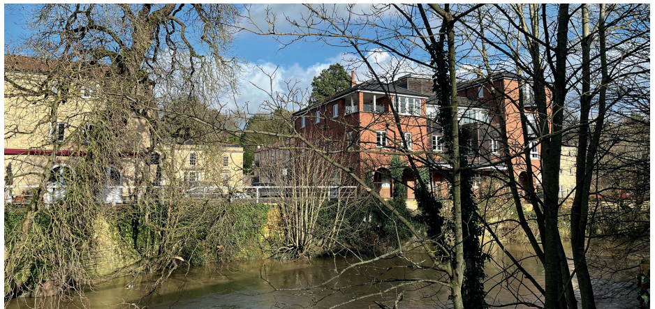
■ A new pedestrian bridge would link the library car park with Kingston Square and Kingston Road
