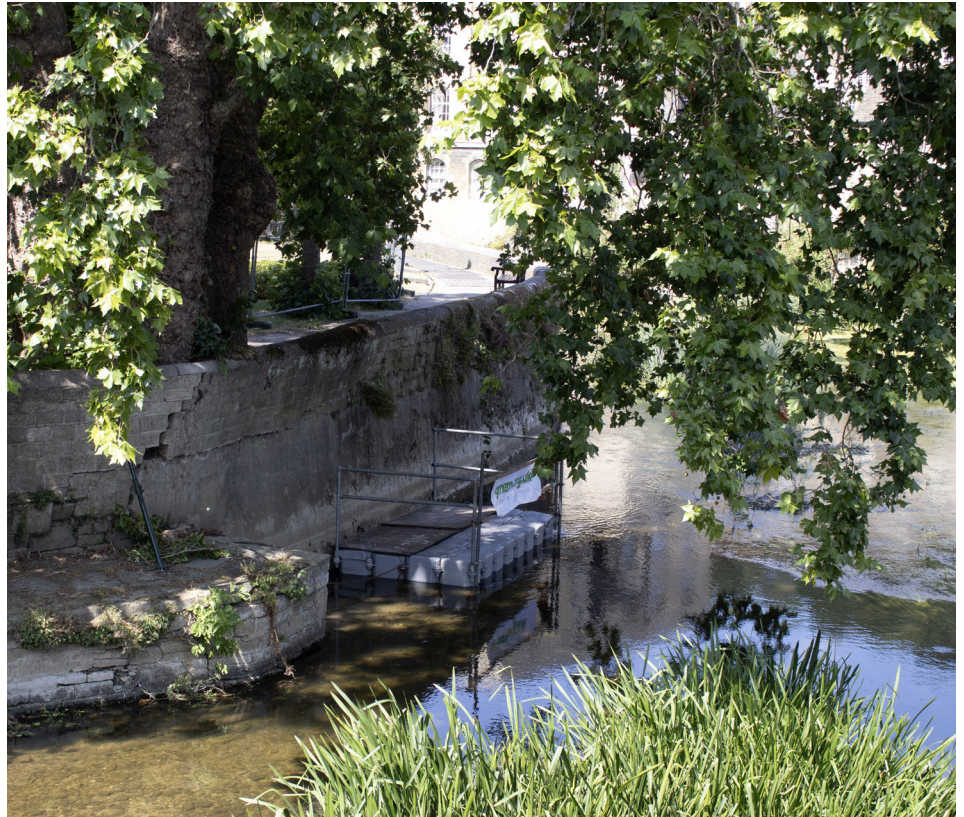
work at the riverside wall at Westbury Garden
