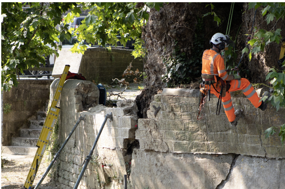
■ contractors working on the wall this spring
